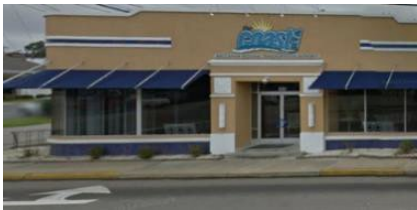
Conway Terminal 1418 Third Avenue Conway, SC
